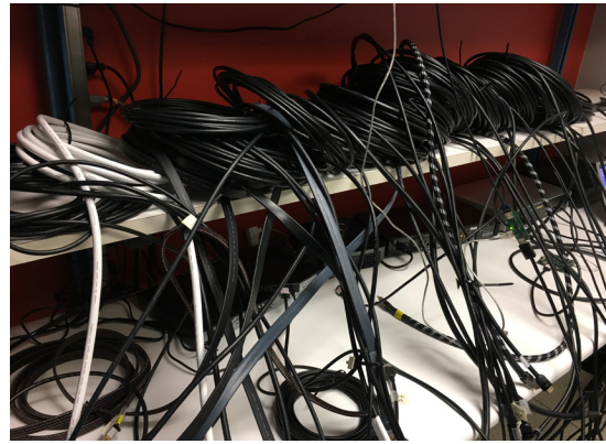
Fig. 7 Long reach UHD cables used in retrofitting test
