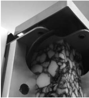
Kabel vom Türelement vom 90° Knoten zur Decke führen Route the cable from the door element from the NOOXS Corner to the ceiling
