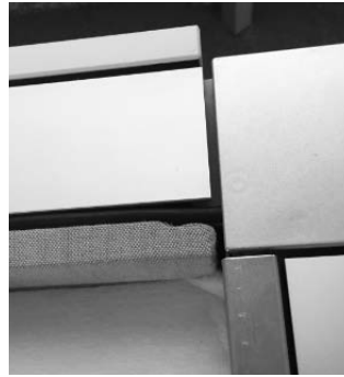
Kabel vom Türelement vom 90° Knoten zur Decke führen Route the cable from the door element from the NOOXS Corner to the ceiling
